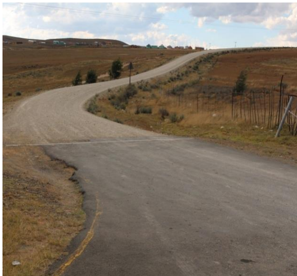
UPPER INDWANA ACCESS ROAD PHASE 1& 2
